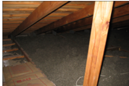
Highest level in attic
